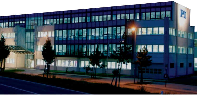
PI headquarters in Karlsruhe
